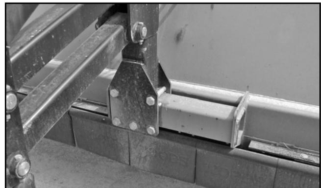
Figure 46. Strut Uprights Installed
