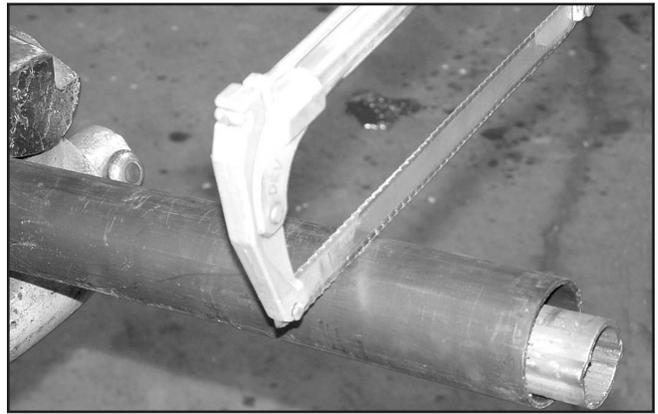
**Figure 7.** Cut Shield
